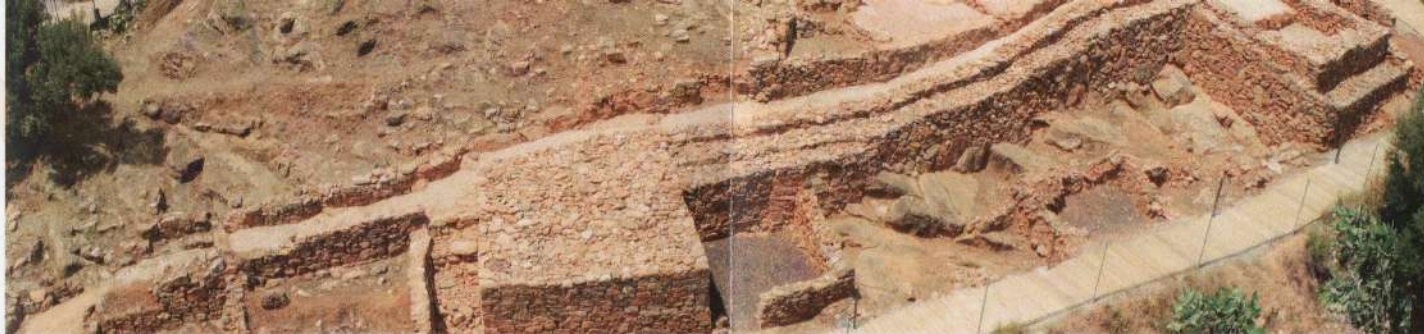
General view of the wall and towers B and A. Picture: José Solà
