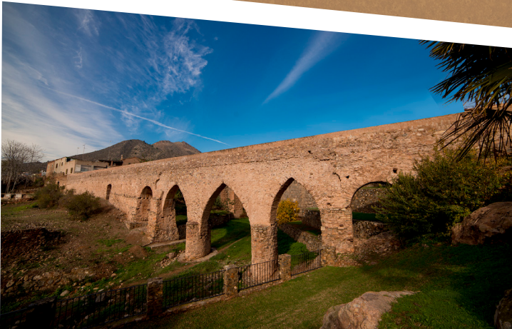
Aqueduct of Sant Josep
